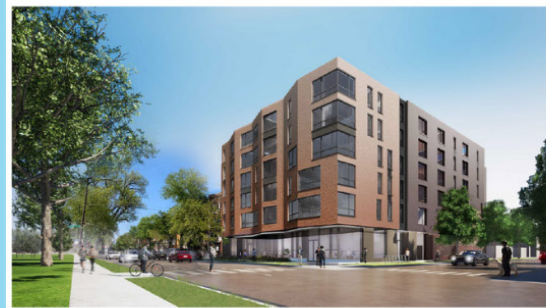
1237 N California 40 Affordable Family Apartments
